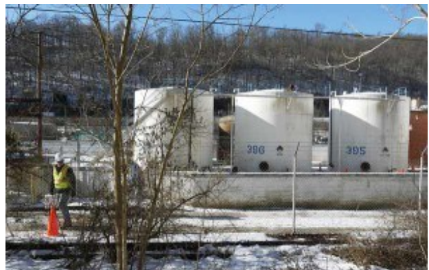
MCHM storage tanks.
