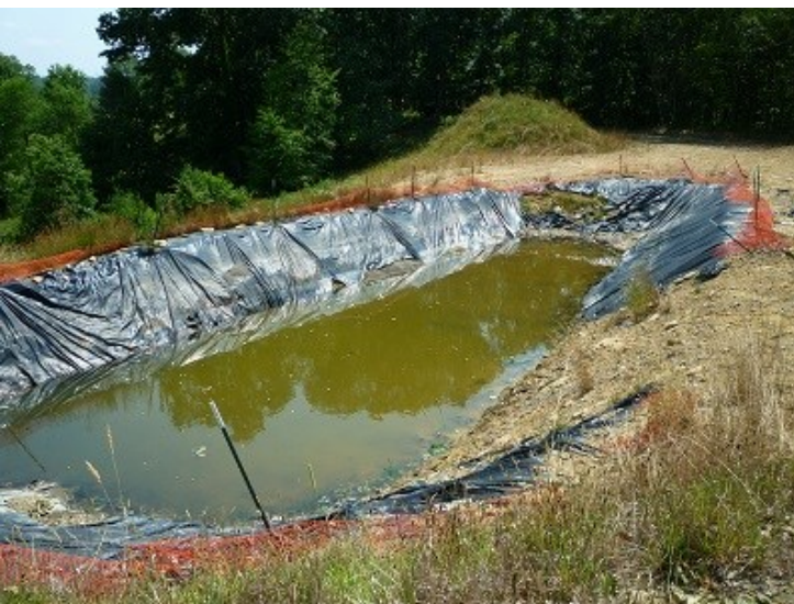
An un-reclaimed drilling waste pit at a well site in Upshur County.
